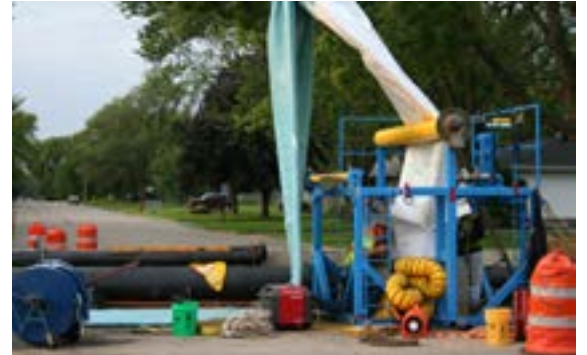
Sewer re-lining process
